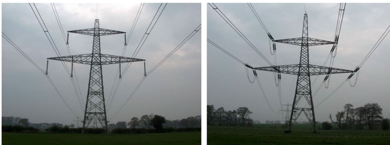
Image 5.14 Typical low height lattice pylon (suspension (left) and tension pylon (right)) 4 (source: Land Use Consultants, 2024)
